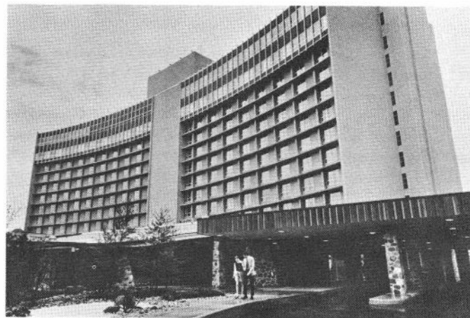
The Arlington Towers, Chicago, Illinois
